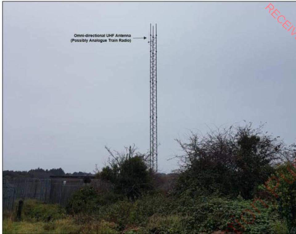
Plate 15-1 Telecoms Mast at Claremorris Train Station
